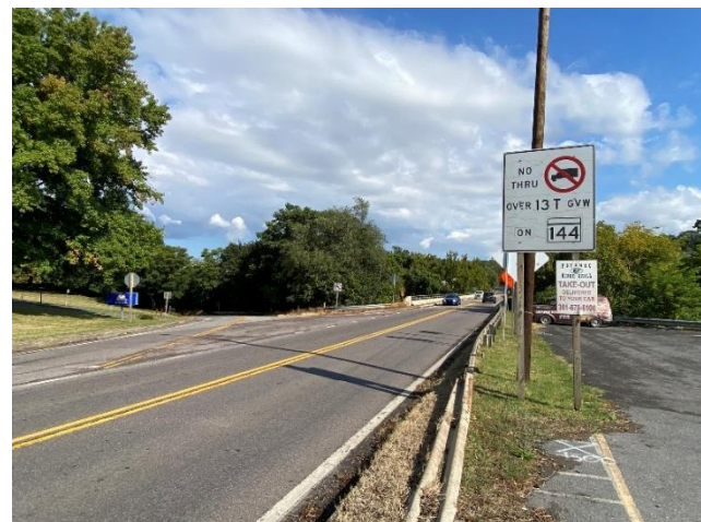
Figure 12 Access to One of the US 522 Bridges with a Weight and Size Restriction Signage for Heavy Trucks
