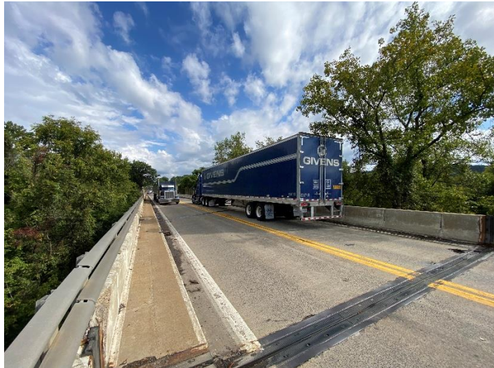
Figure 9 Trucks Navigating the Tight Two-Lane Cross Section on One of the US 522 bridges
