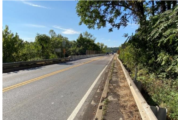
Figure 4 US 522 Bridge over the Potomac River
