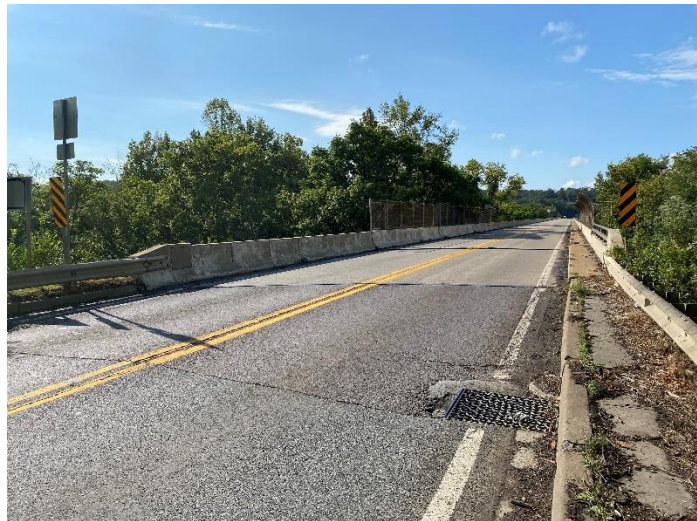
Figure 6 Elevation View of One of the US 522 Bridges
