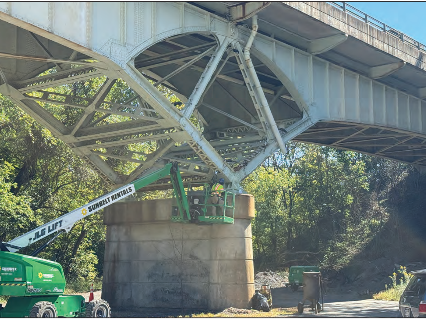
Work began last week on the superstructure of the U.S. 522 bridge crossing the Potomac River and train tracks and into Hancock. The steel work comes after the bridge was classified by the Federal Highway Administration as being in “poor condition” with sub- and superstructure ratings of four. The substructure work was completed this past July. While workers are making repairs to the superstructure of the bridge, traffic going across will be subjected to one lane of traffic Mondays through Fridays from 9 a.m. to 3 p.m. Work should be completed by mid October.
