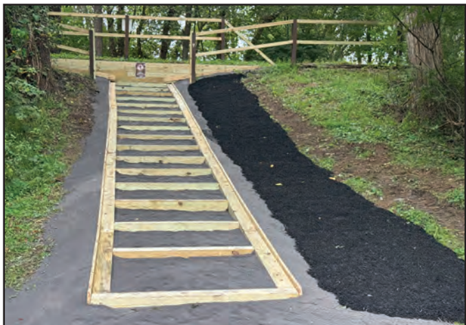
REM recently completed the stairs from Joseph Hancock Park to the Western Maryland Rail Trail after being awarded the contract in June of this year. The wood for the stairs is pressure treated, stone dust was laid, and mulch put down to dress up the area and give a place for bicycle riders to bring their bike up the steps.
