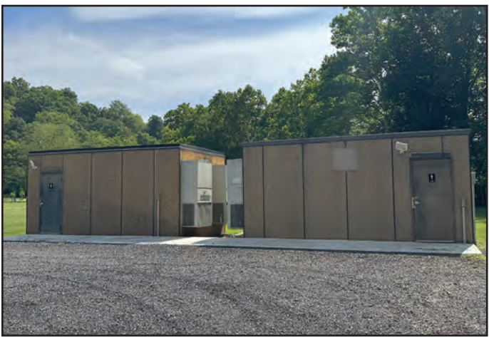
Town officials also approved the purchase for new heating and air conditioning units at the restrooms by the Kirkwood Park pavilion.
