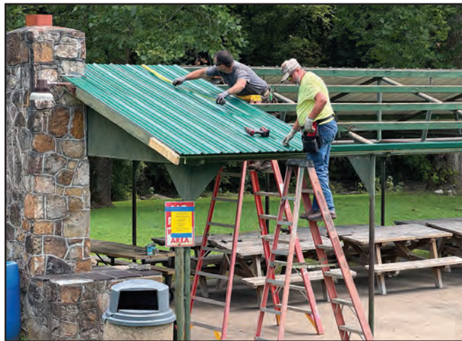
A crew from Norris Building Contractors were in Widmeyer Park on Monday, August 24, working on the pavilion roofs after being awarded the contract to do so on the pavilions in Widmeyer Park and Joseph Hancock Park.
