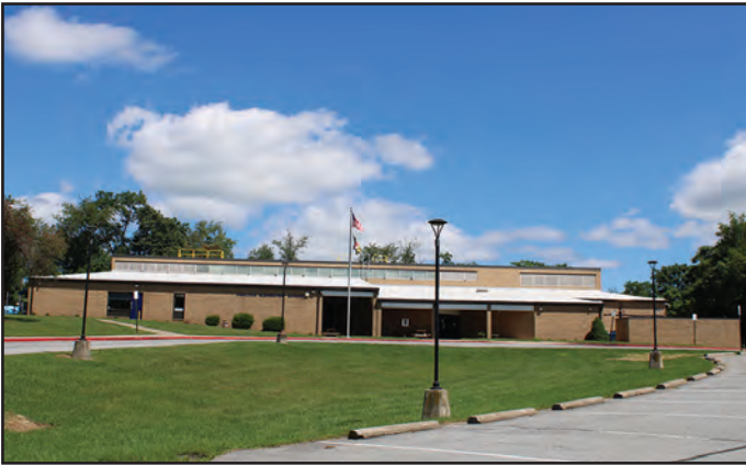
Hancock Elementary School
