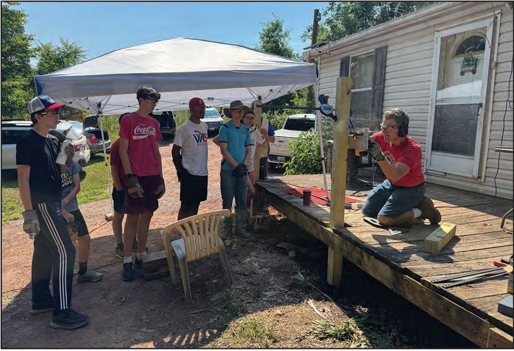
Jim Mullkin demonstrates to the work team from Camp Joy how to properly use the saw to make sure the railing post is level when it’s cut.
