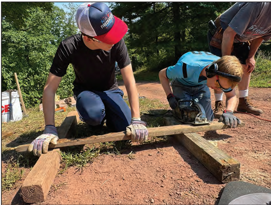
Ned Flugge holds the board as Nate Kovacs saws the wood to be used for a deck at a worksite in Berkeley Springs for Camp Joy.
