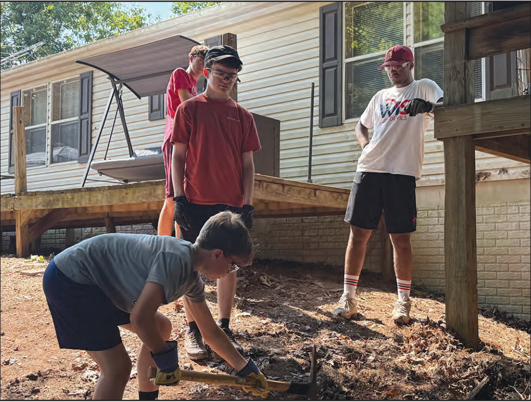
Desmond Ryan digs the earth to make a setting for a stand that will hold the leg of a deck. John Tollison and Carter Samuel were helping to make sure the hole was level.
