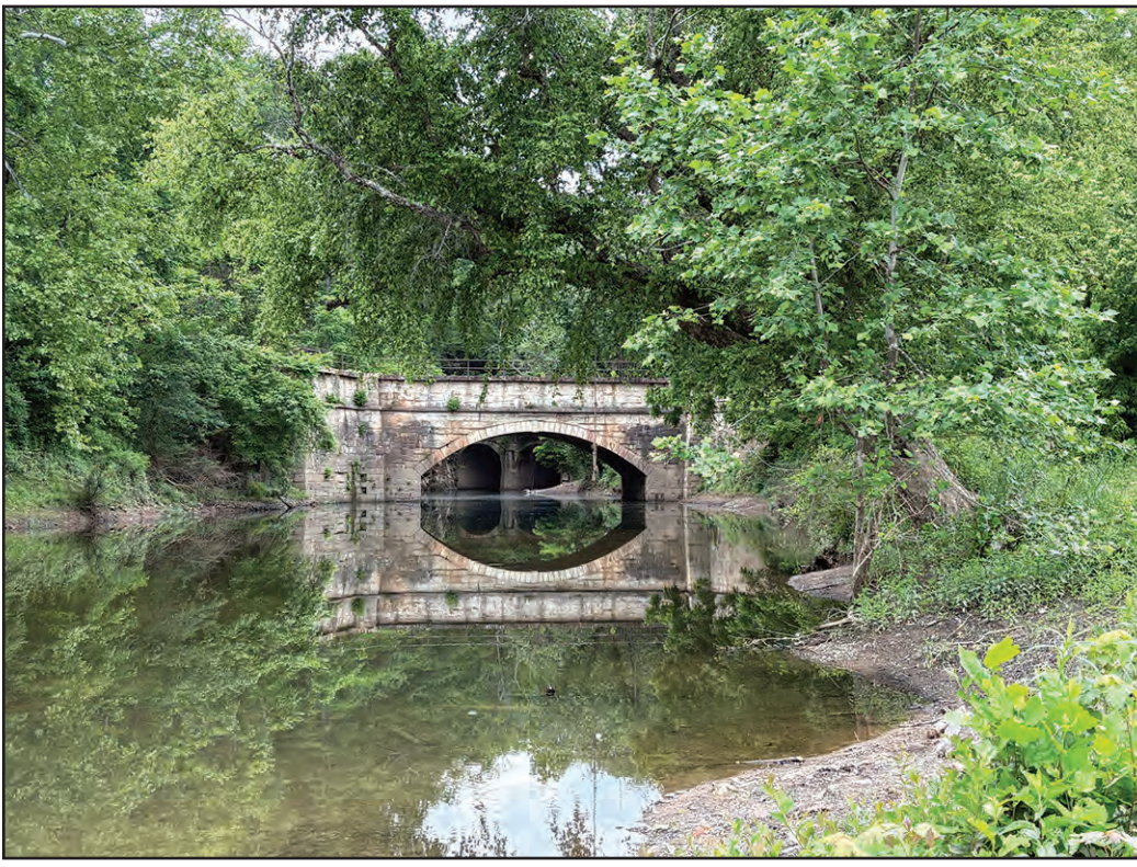
Dating back to the days of the C&O Canal, the Fifteen Mile Creek Aqueduct still stands in Little Orleans. It was built sometime between 1838 and 1850 of hard flint stone cut from Siding Hill on the West Virginia side of the Potomac River. Photographer Justin Mellott took this portrait of the structure during a recent visit to the area, where the Western Maryland Rail Trail and C&O Canal Towpath are in close proximity, just where Fifteenmile Creek empties into the Potomac River.
