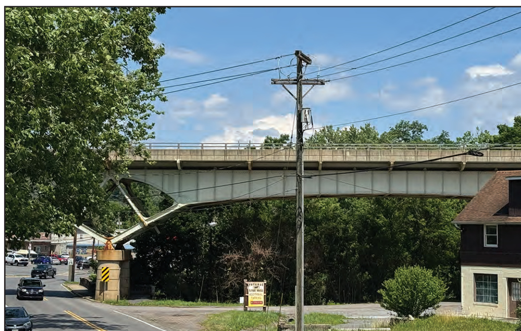
Hancock's bridge over Main Street and Little Tonoloway Creek.
