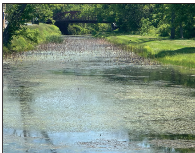
The condition of the canal was among concerns brought up to council members.
